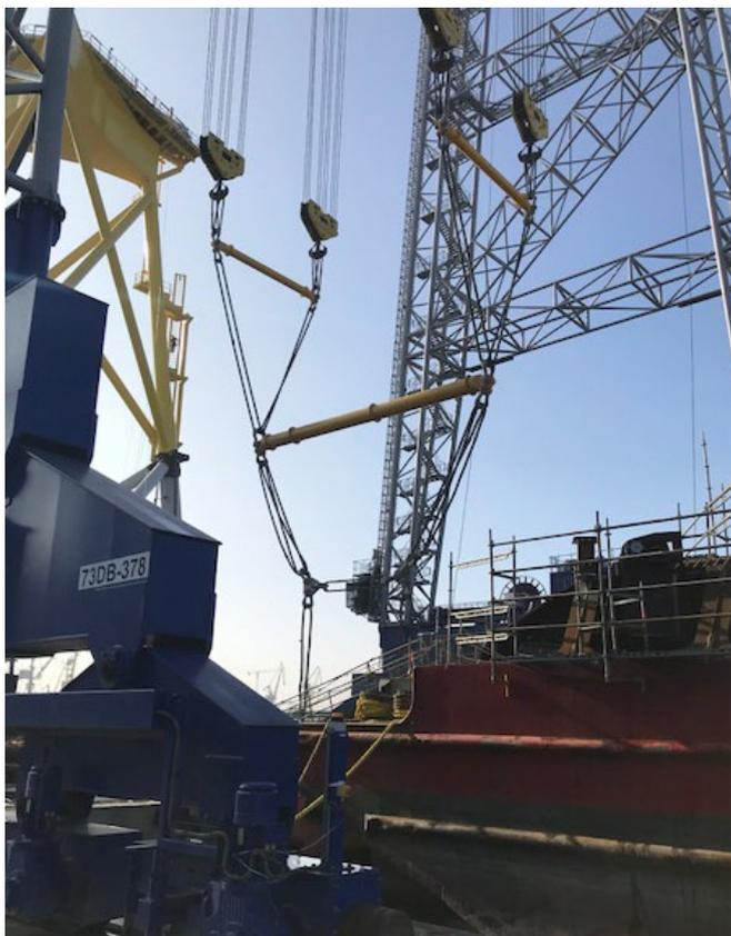
Baker added: "Modulift spreader beams are put into compression when loaded so another beam wouldn't have been suitable at the bottom of the rig between the delta plates because the forces applied are tensile rather than compressive. A wire rope grommet acted as a tie sling between the delta plates and created the vertical sling angle for the bottommost slings in the rig."
