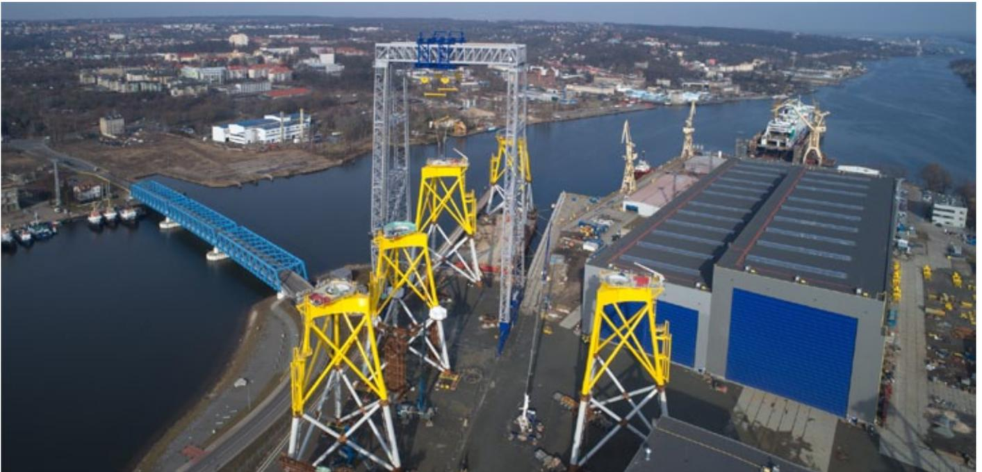
Modulift has supplied two large spreader beams to complete a rig that will lift 20 wind farm jacket foundations onto vessels at ST3 Offshore's dockside location in Szczecin, Poland, close to the country's northwestern border with Germany. The jackets are bound for Cuxhaven and will eventually be installed at the Borkum Riffgrund 2 offshore wind farm.
