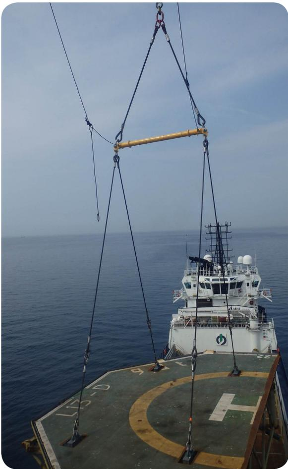
Different rigging equipment was used with each spreader beam. Above the MOD 110H was a two-leg, 7m-long sling made from 90mm diameter wire rope, while beneath the beam were two two-leg, 16m-long slings made from 64mm diameter wire rope. Above the MOD 110, a two-leg, 8m-long, 64mm sling combined with a pair of two-leg, 16m-long, 56mm slings. All were utilised at 30 degrees.
