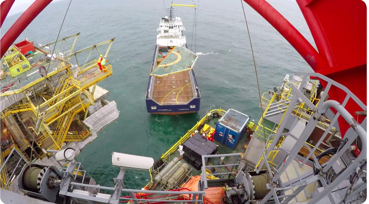
Certex (UK) used two modified spreader beams from Modulift's heavy, off-the-shelf range to lift two none identical halves of a helipad onto a vessel from a gas rig in the Dutch Sector of the North Sea recently. The site was approximately 70 miles off the Danish coast.
