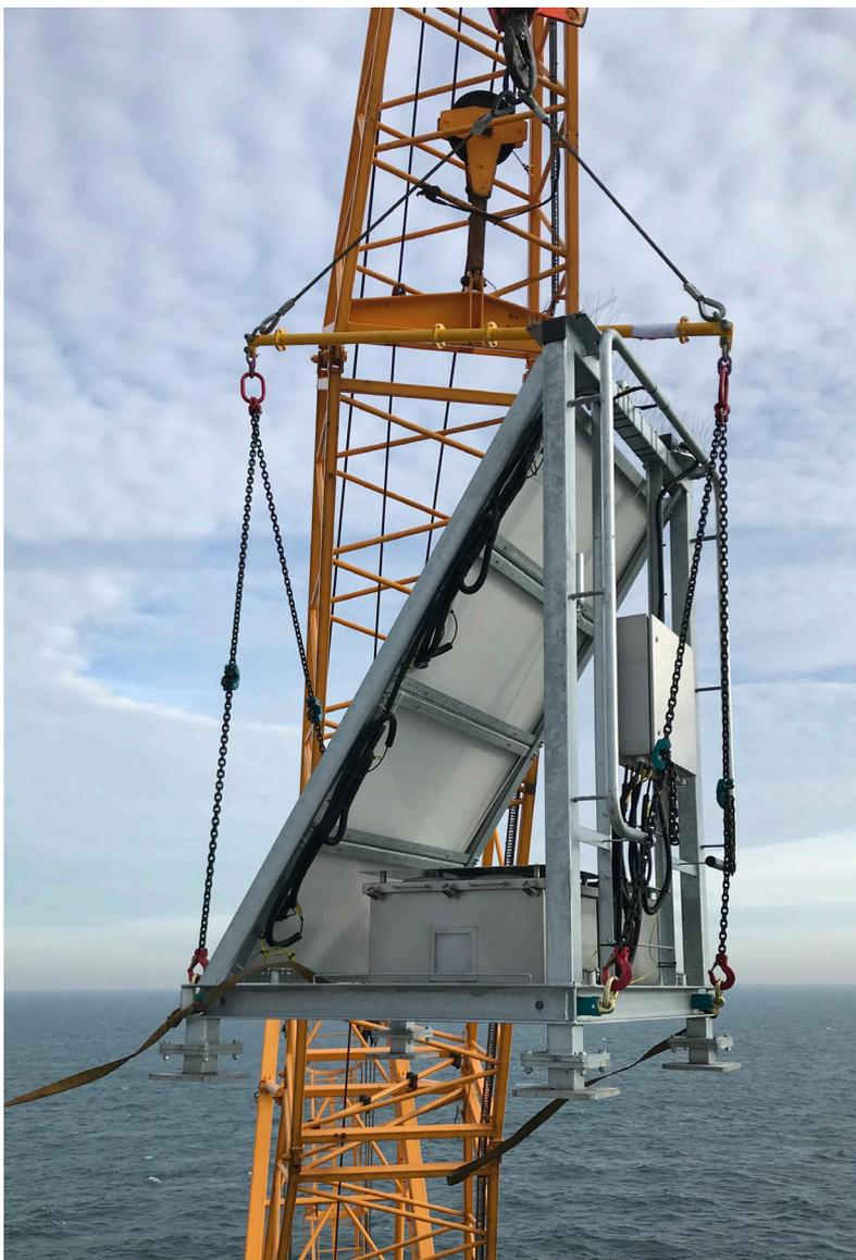
A 6t capacity spreader beam was the linchpin in lifting navigation skids onto offshore structures that guide vessel traffic and helicopters operating in Dutch waters of the North Sea. Centre of gravity was a principle area of concern in each lift due to load dimensions.
