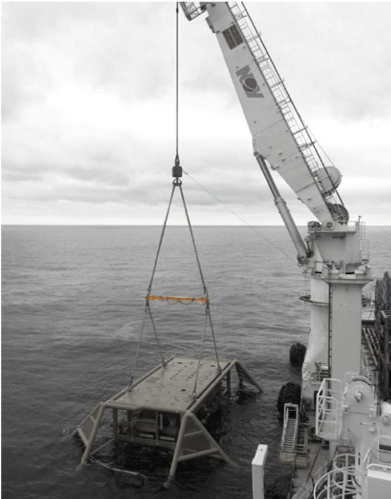
Below-the-hook equipment manufacturer Modulift recently refurbished two subsea spreader beams for a major subsea installation contractor before they were used to lift 260t and 280t manifolds for a field development offshore Libya.
